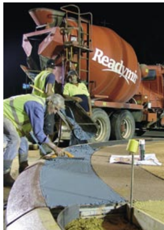
Installation of work by Lance Chadd, Busselton entry upgrade, 2007
